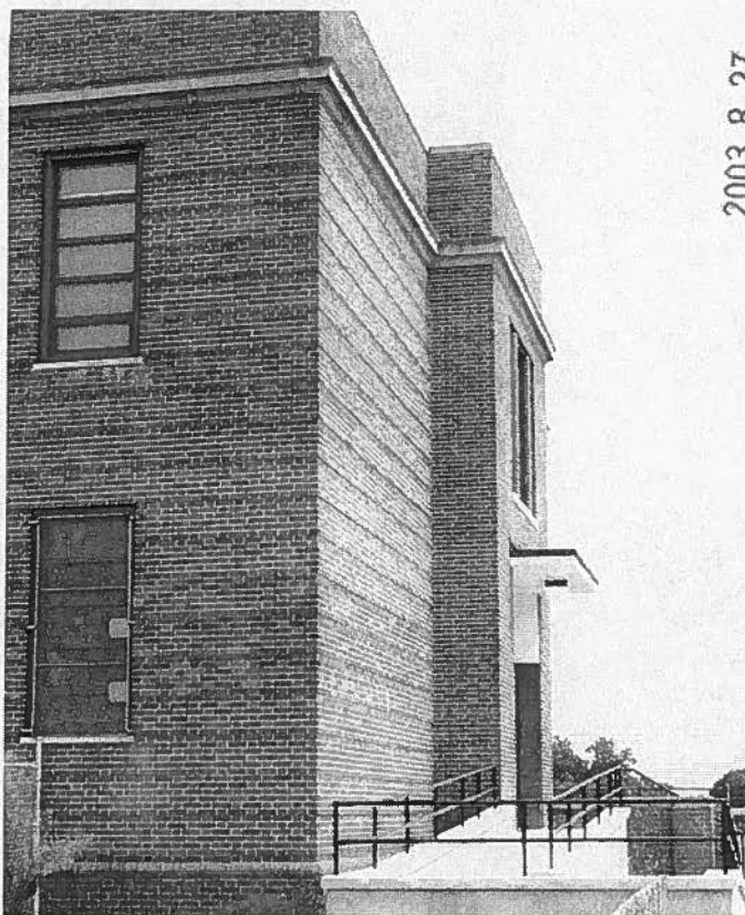
Cherry Hill Elementary School showing brick banding on the end bays.
