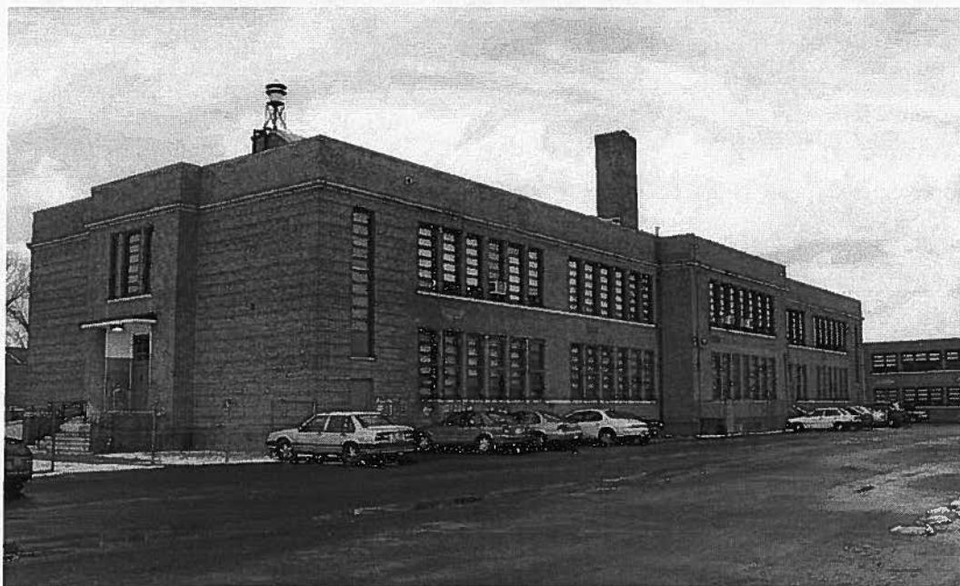
Rear and side facades, Cherry Hill Elementary School.
